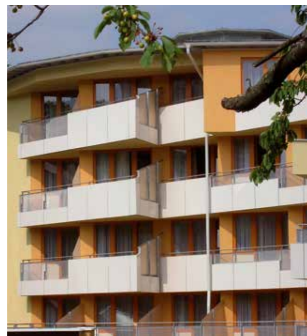
Visible fixing to the balustrade supports - continuous board
