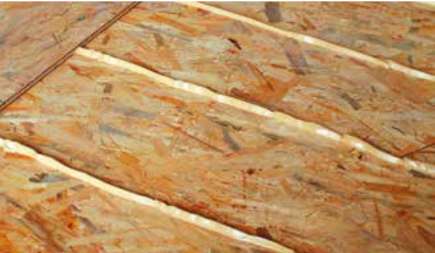
Image13: Gluing OSB boards with gun
